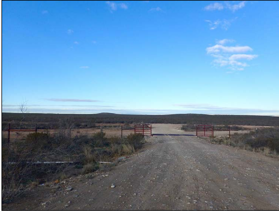
Figure 3.12. KOP 5 facing west toward the China Draw Substation.
